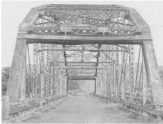
Figure 1.3 Uniform corrosion (atmospheric attack) of a steel bridge.
