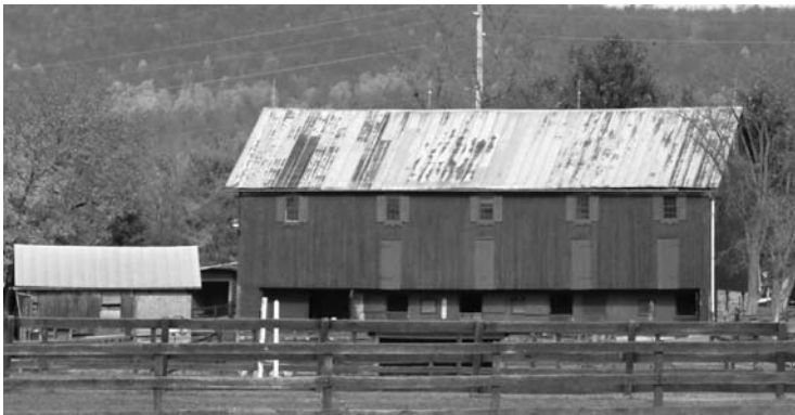
Fig. 5.8 The corrosion of a galvanized roof in the natural atmosphere. When the protective zinc coating is breached, the underlying steel eventually suffers corrosion
