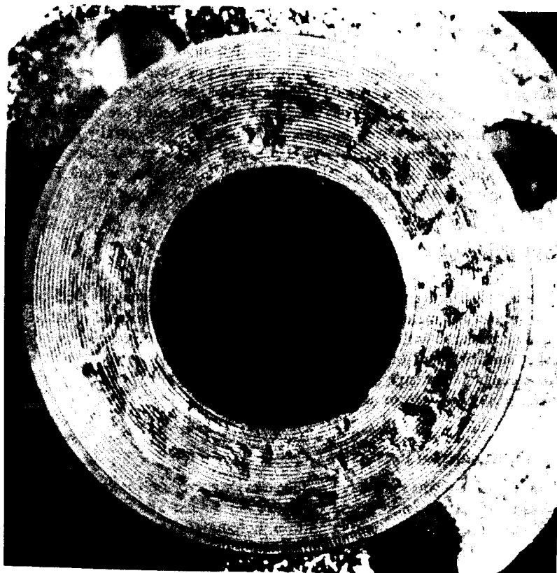
Figure 3-8 Gasket (crevice) corrosion on a large stainless steel pipe flange (E. V. Kunkel.)
