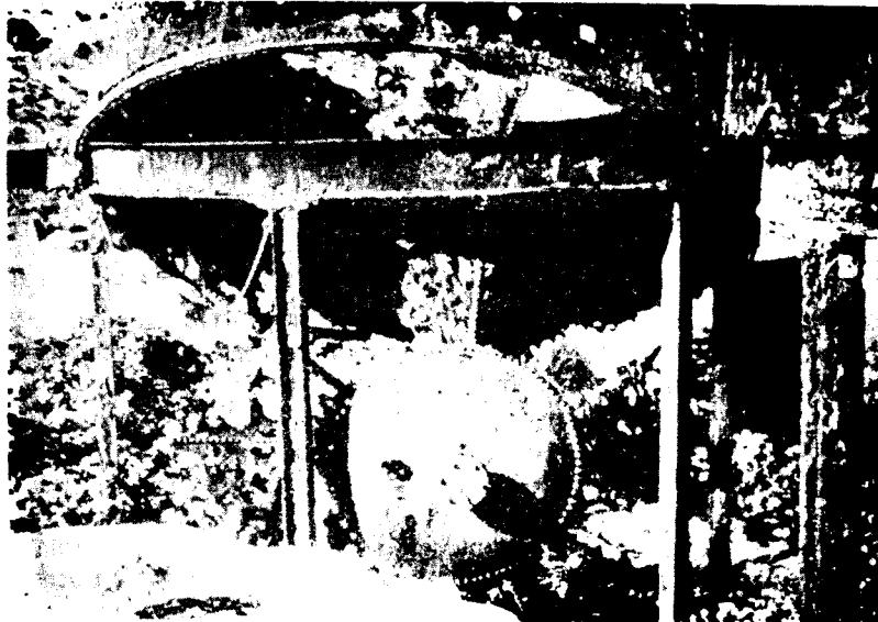
Figure 3-1 Rusting of abandoned steel tank.
